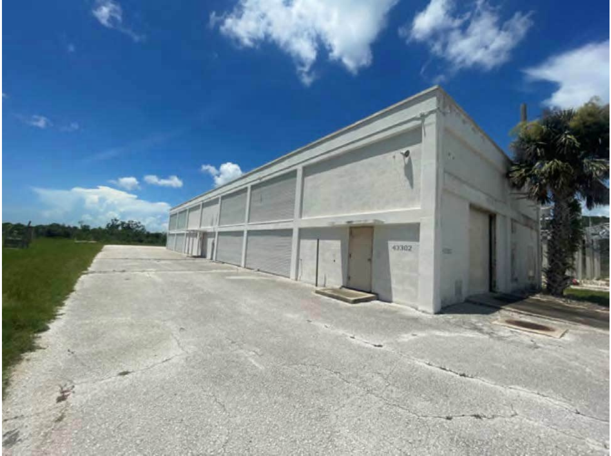
Photograph 1. Delta IV Warehouse, Facility 43302 (FMSF No. BR4030) from the parking lot with the electrical substation at the rear, facing southwest.
