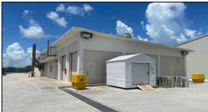
Photograph 9. Delta IV Precision Clean Lab, Facility 43400 (FMSF No. BR04029), facing southwest.
