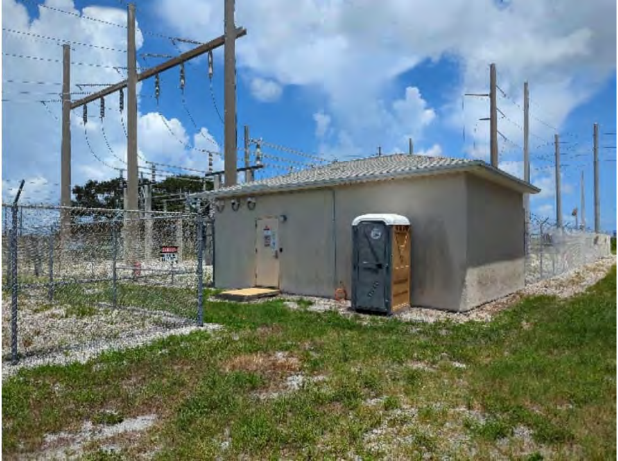
Photograph 1. FPL Substation Building, Facility 43311 (previously unrecorded), with a porta-potty in front and an electrical substation in the background, facing northwest.
