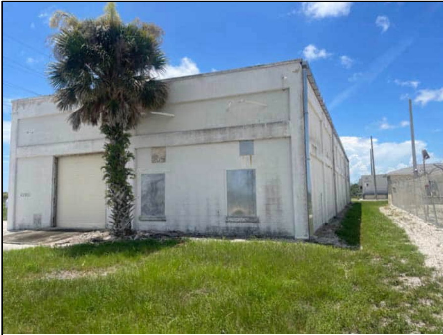
Photograph 11. Delta IV Warehouse, Facility 43302 (FMSF No. BR4030), facing east.
