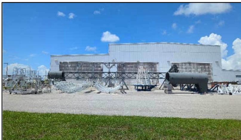
Photograph 5. Horizontal Integration Facility, Facility 38200, facing south.
