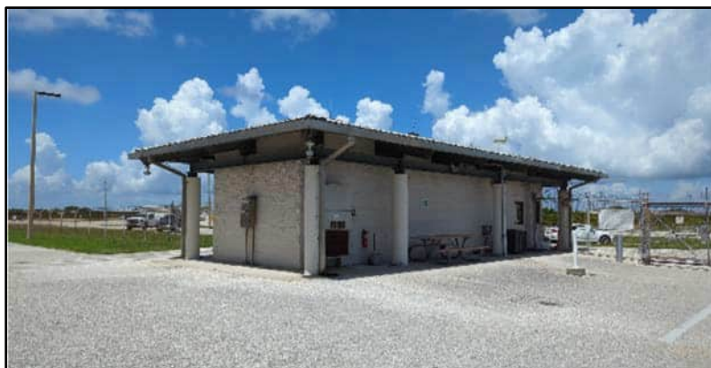
Photograph 6. Security Entry Control Building, Facility 38201, facing west.
