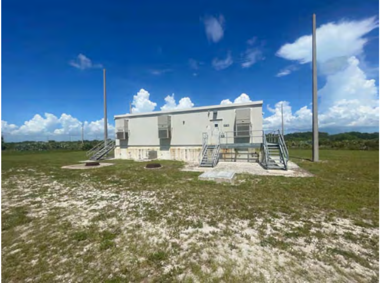
Photograph 1. The Electrical Switch Station, Facility No. 38015 (previously unrecorded) from Beach Road, facing northwest.
