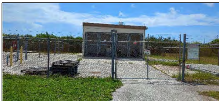
Photograph 10. Hazardous Storage Facility 38316, facing east.
