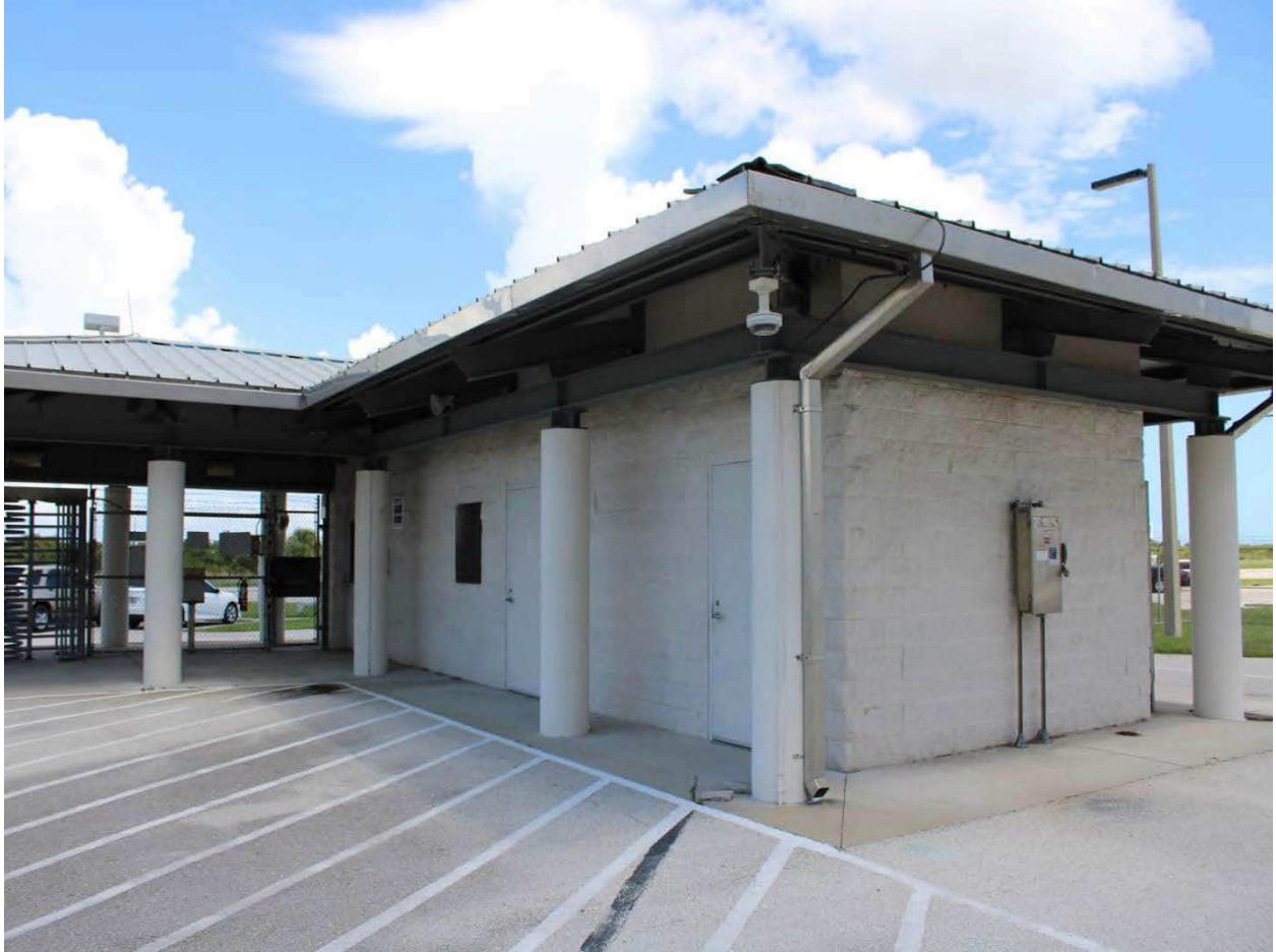
Photograph 1. Security Entry Control Building, Facility 38201 (previously unrecorded) from Horizontal Integration Facility, Facility 38200 parking area to Beach Road, facing northwest.
