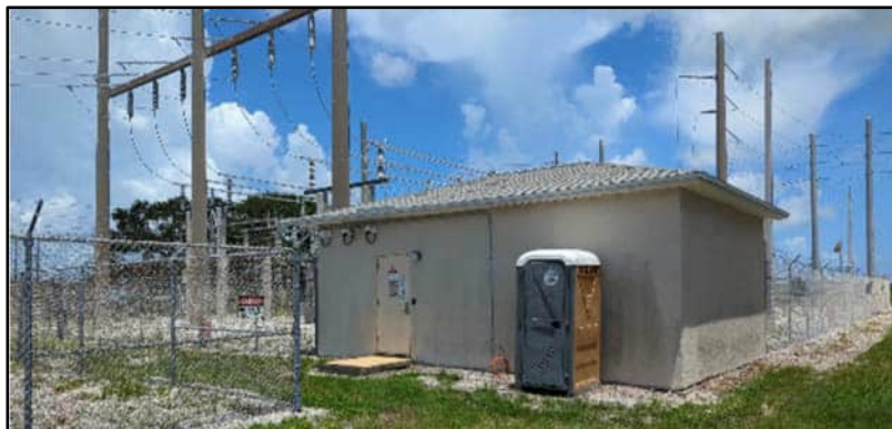
Photograph 12. FPL Substation Building, Facility 43311, facing north.
