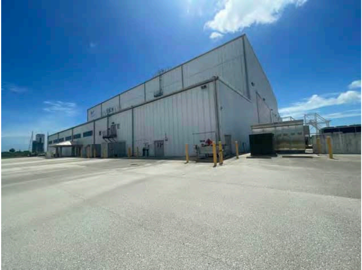
Photograph 1. The Horizontal Integration Facility, Facility 38200 (previously unrecorded) from Beach Road with SLC-37 in distance, facing northeast.
