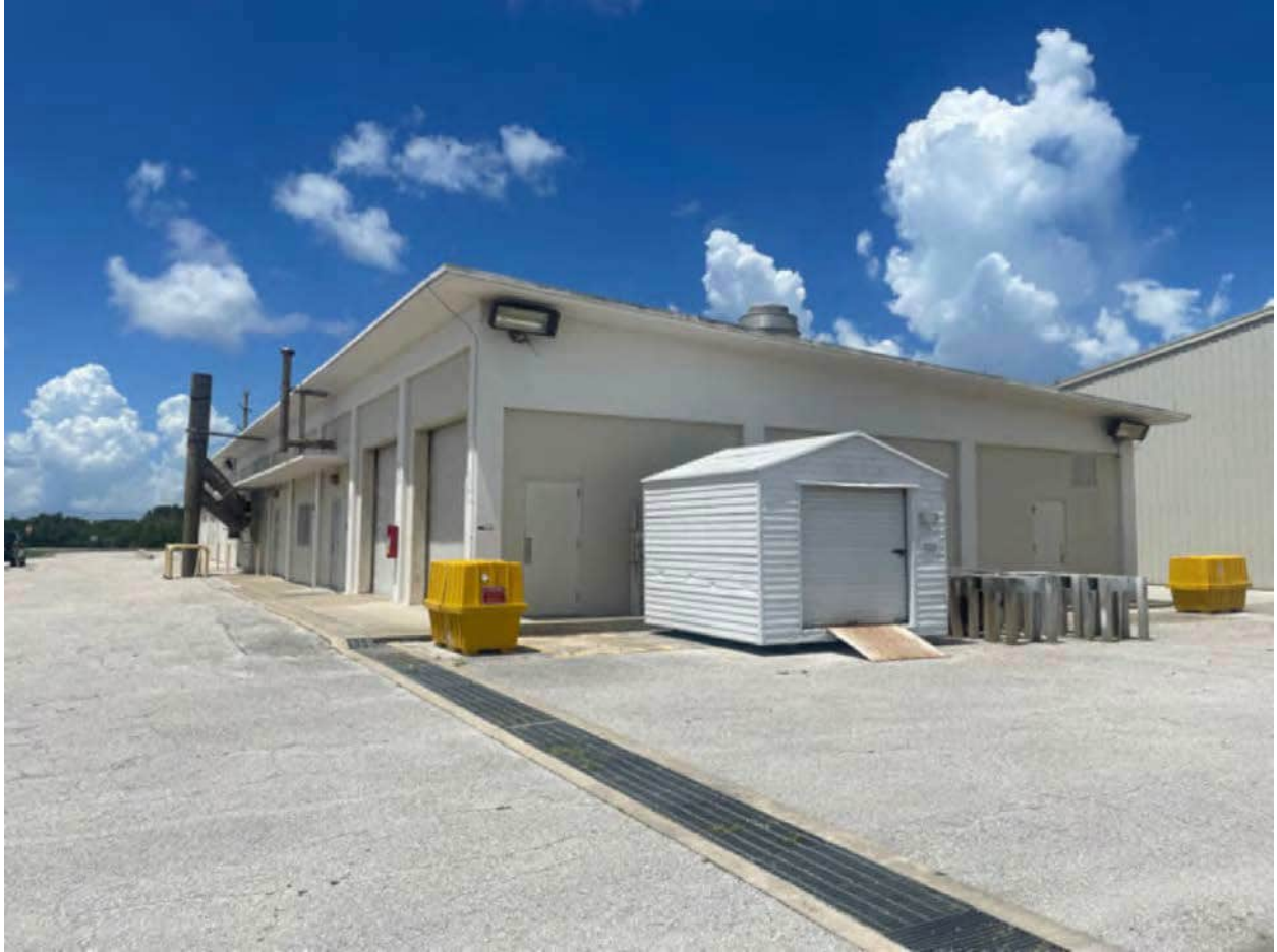
Photograph 1. The Delta IV Precision Clean Lab, Facility 43400 (FMSF No. BR4029), from the parking lot, facing southwest.
