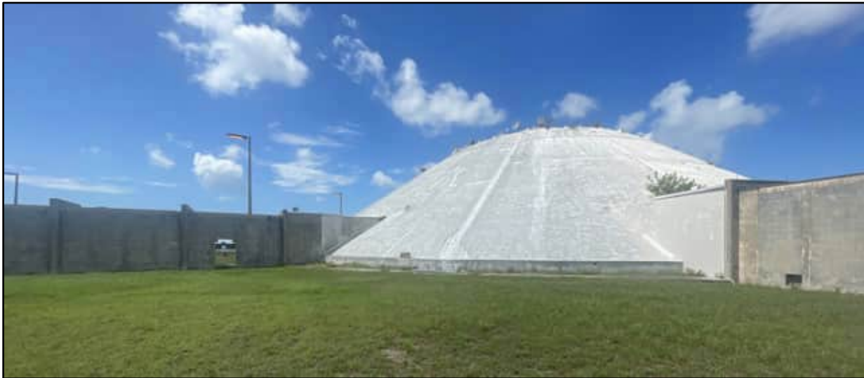
Photograph 2. Built in 1962, the LCC (FMSF No. BR02790) and Cableways (FMSF. No. BR02334) within SLC-37, facing southwest.
